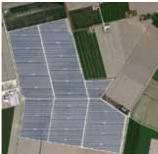
34,8 MWp PHOTOVOLTAIC PLANT
