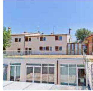
60 kW GEOTHERMAL PLANT
